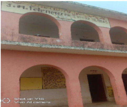
Polling Station Front View
