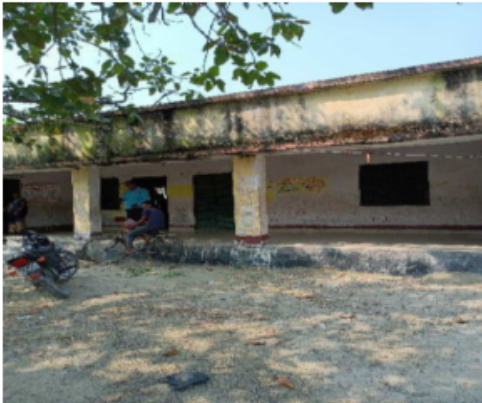
Polling Station Front View
