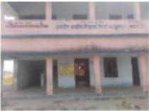
Polling Station Front View
